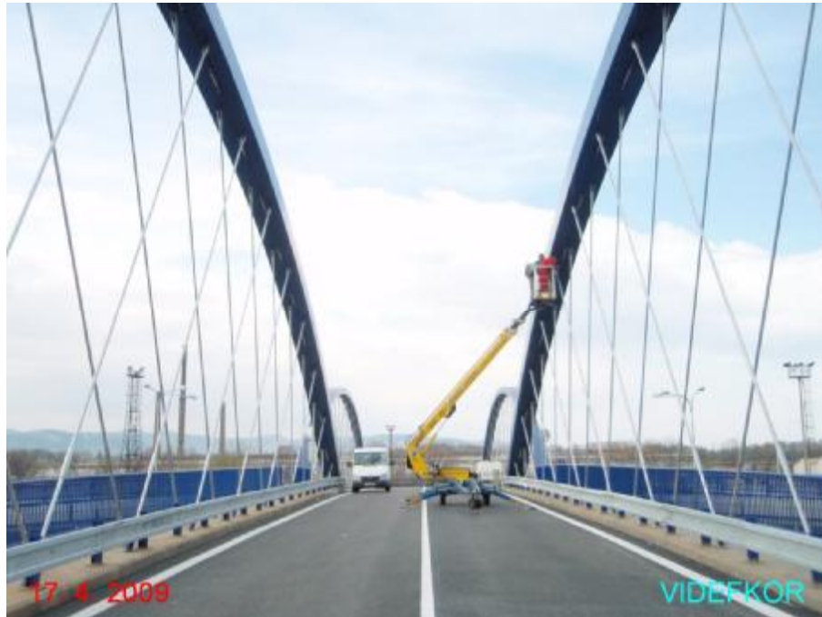
The road bridge in Třinec – Baliny
