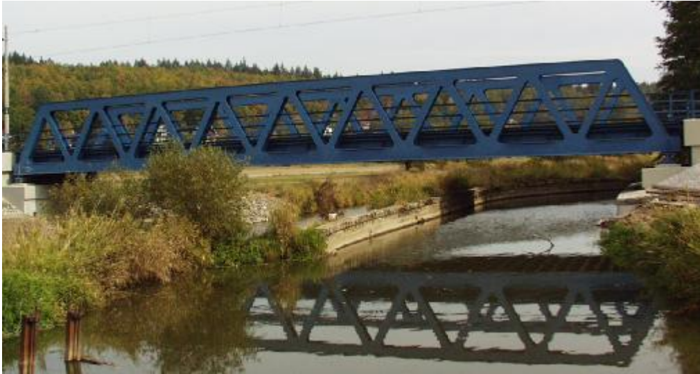
The railway bridge in Heřmaň
