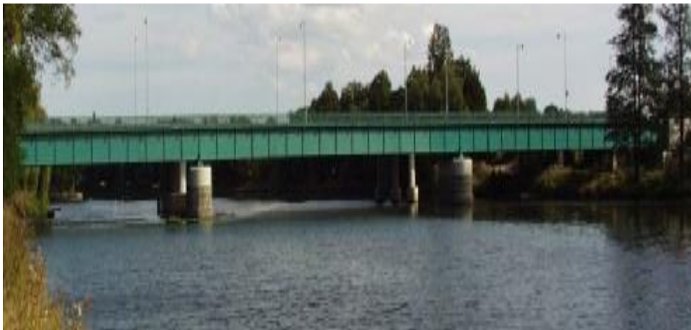
The railway bridge in Písek
