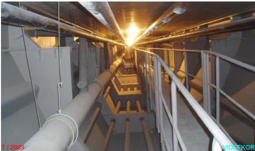
The inside coating of highway bridge over Odra river in Ostrava.
