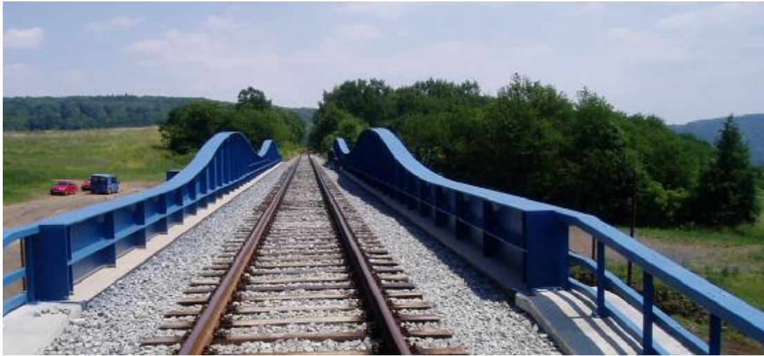
The railway bridge in Varvažov
